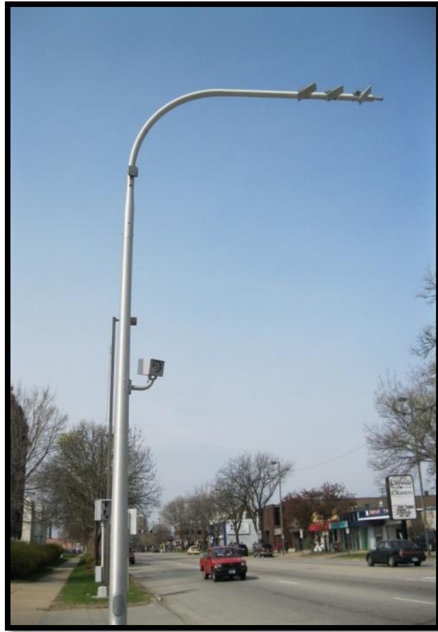
Figure 7: Mast arm and RF Antenna Set up
